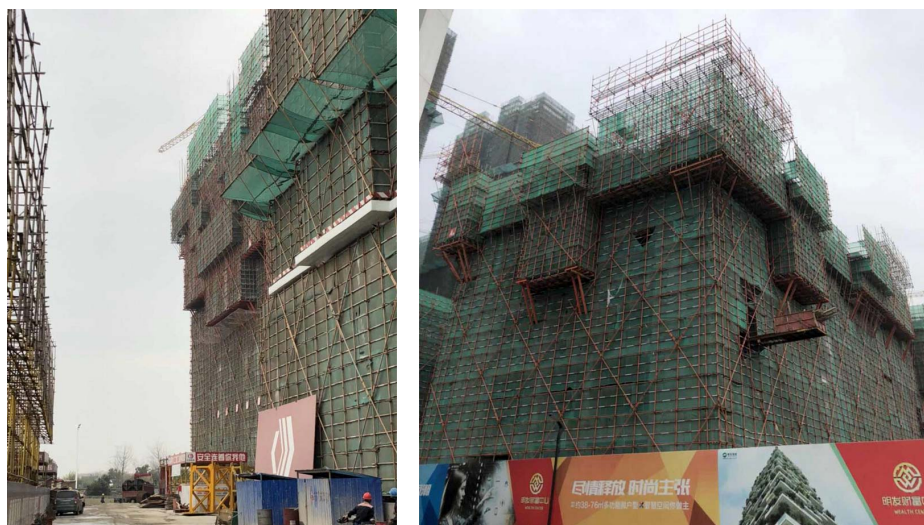
Figure 18: Photographs of the "Green Towers" construction project in Nanjing, Pukou's District
